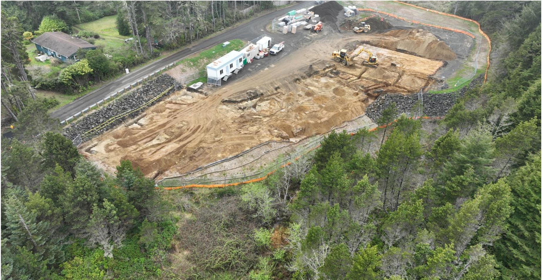
UCMF Construction - Underway
