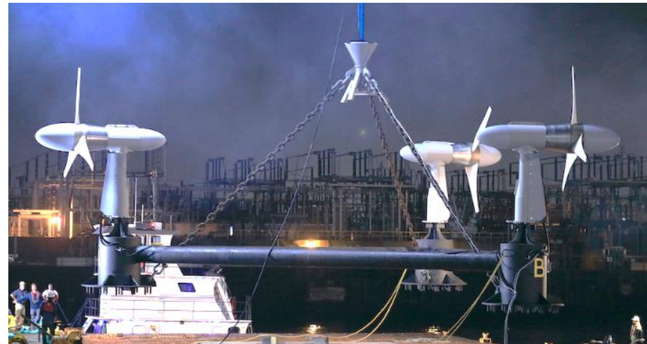
Deploying three turbines significantly lowers the on-water work time and CAPEX and OPEX for installation and O&M, while maintaining optimal hydrodynamic performance
