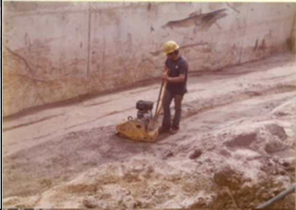
Construction Photographs of Filter Placement around the Conduit
