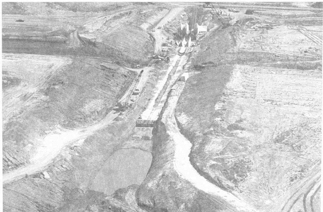
Construction Photograph of Outlet Works Excavation
