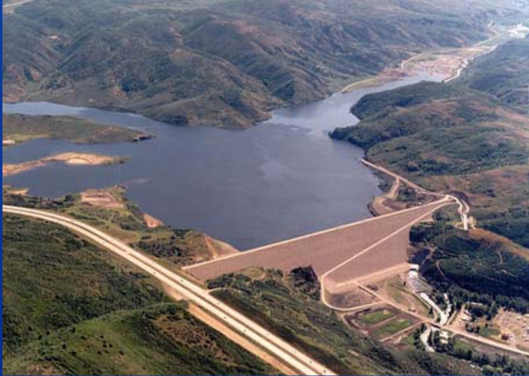
Jordanelle Dam and Power Plant
