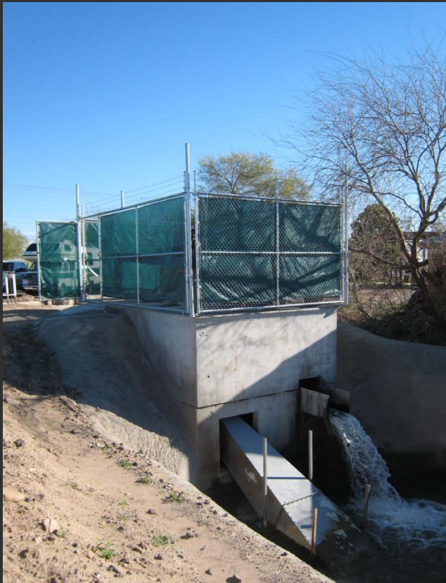
Security fence installed around powerhouse
