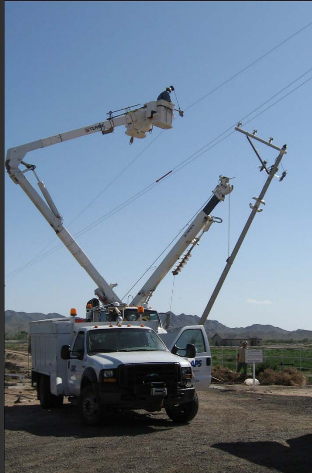
Installation of the pole and transformer
