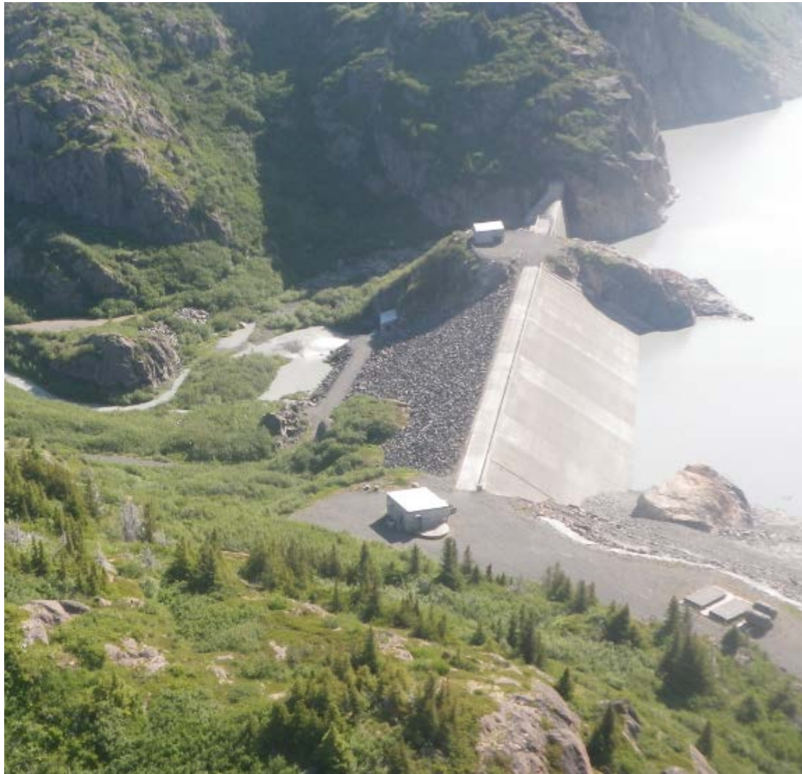
Example of Concrete Faced Rockfilled Dam
